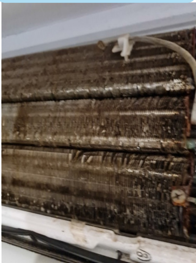
COILS BEFORE UV-C
